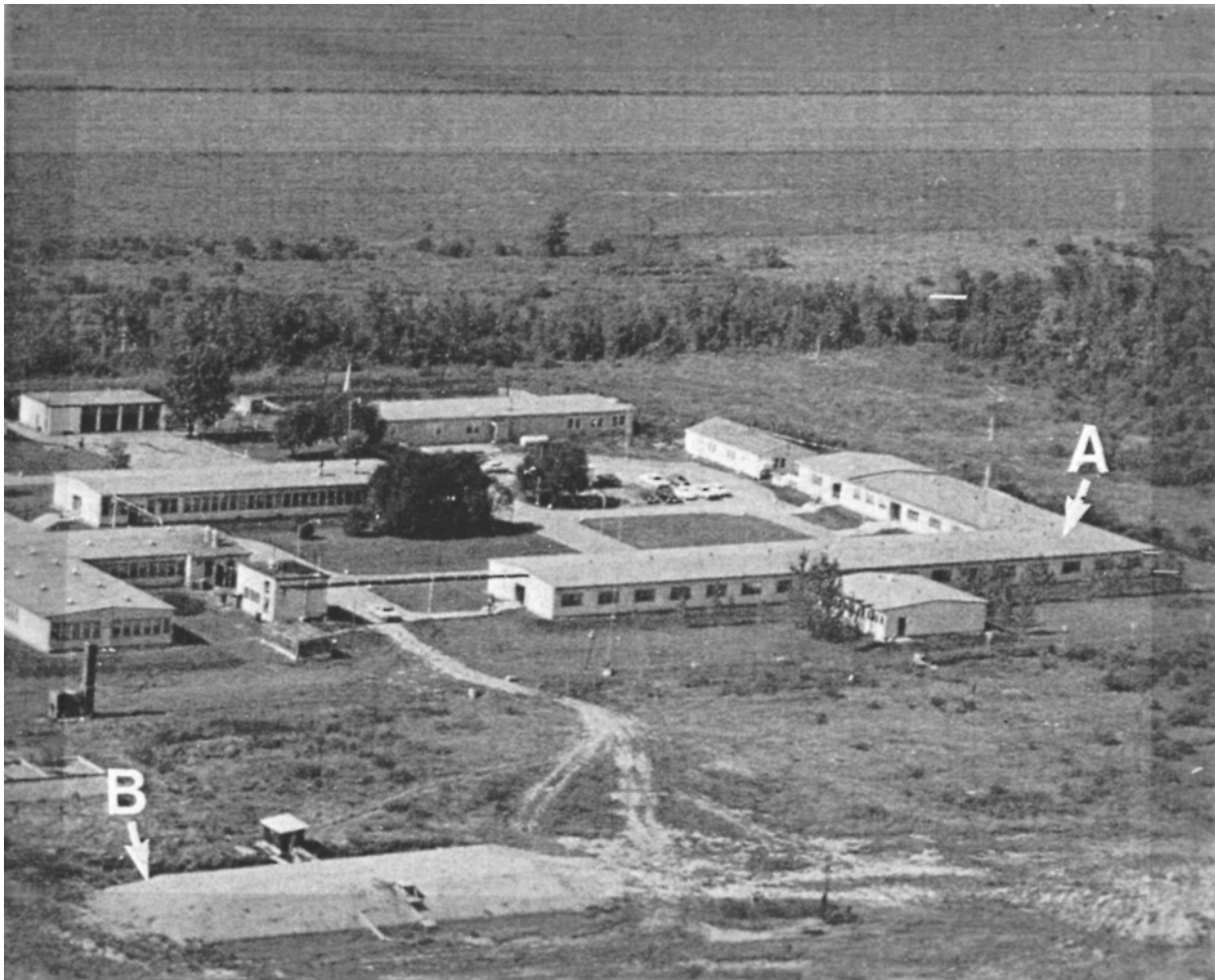
Fig. 3. Aerial view of test fill (B) and accommodation building (A) at Gloucester (after Crawford and Bozozuk 1990).
